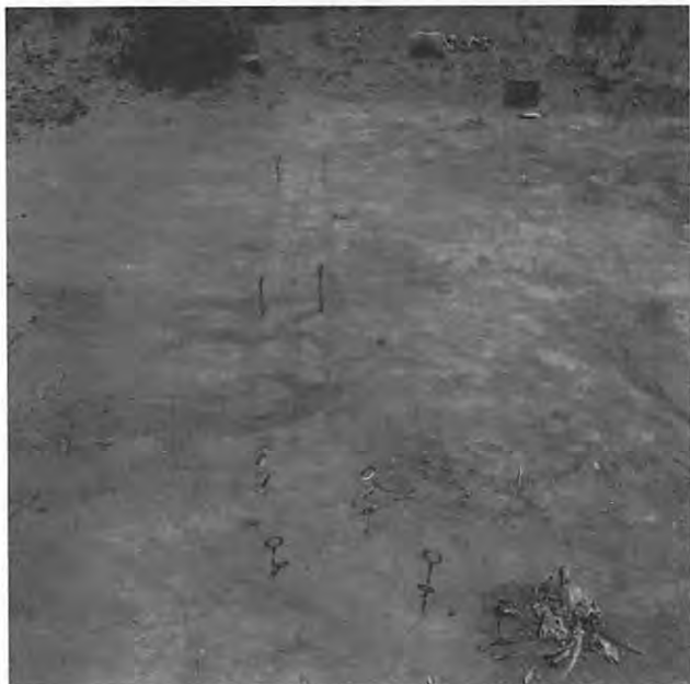
Figure 50. View north of exposed west wall of Structure B.
